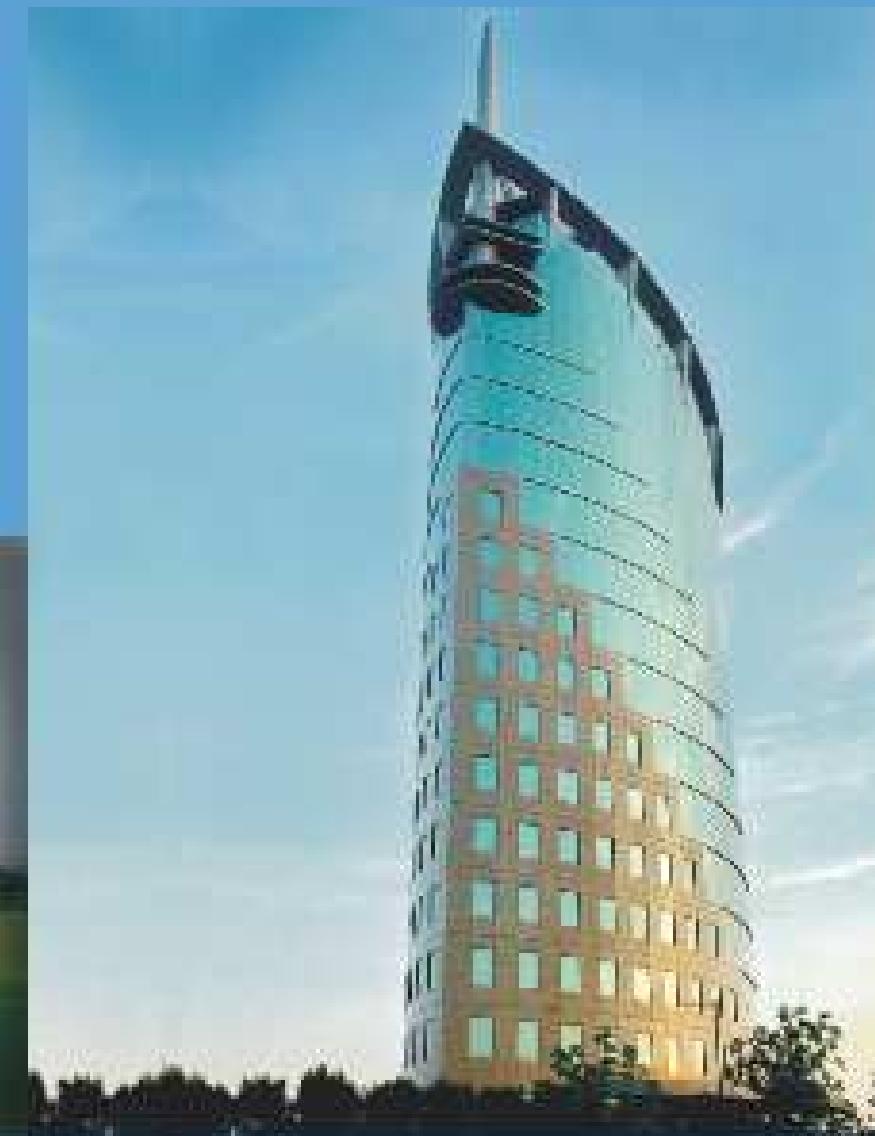
Gateway Tower, Gurgaon
